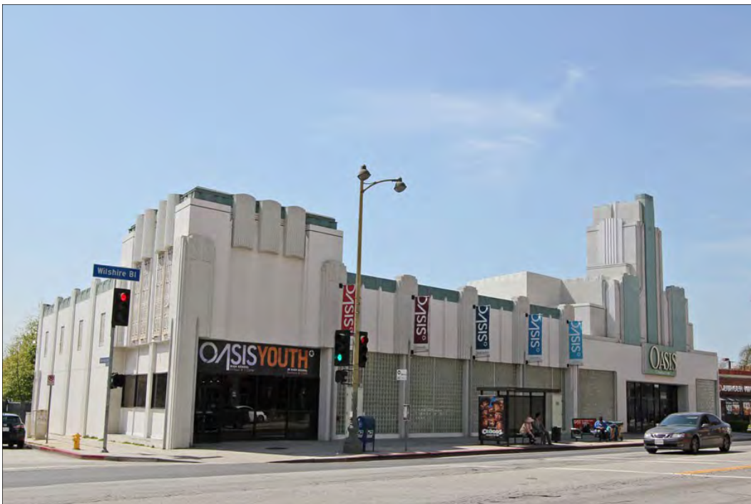
Figure 2: North elevation (right) and east elevation (left), view southwest (Chattel, 2013)
