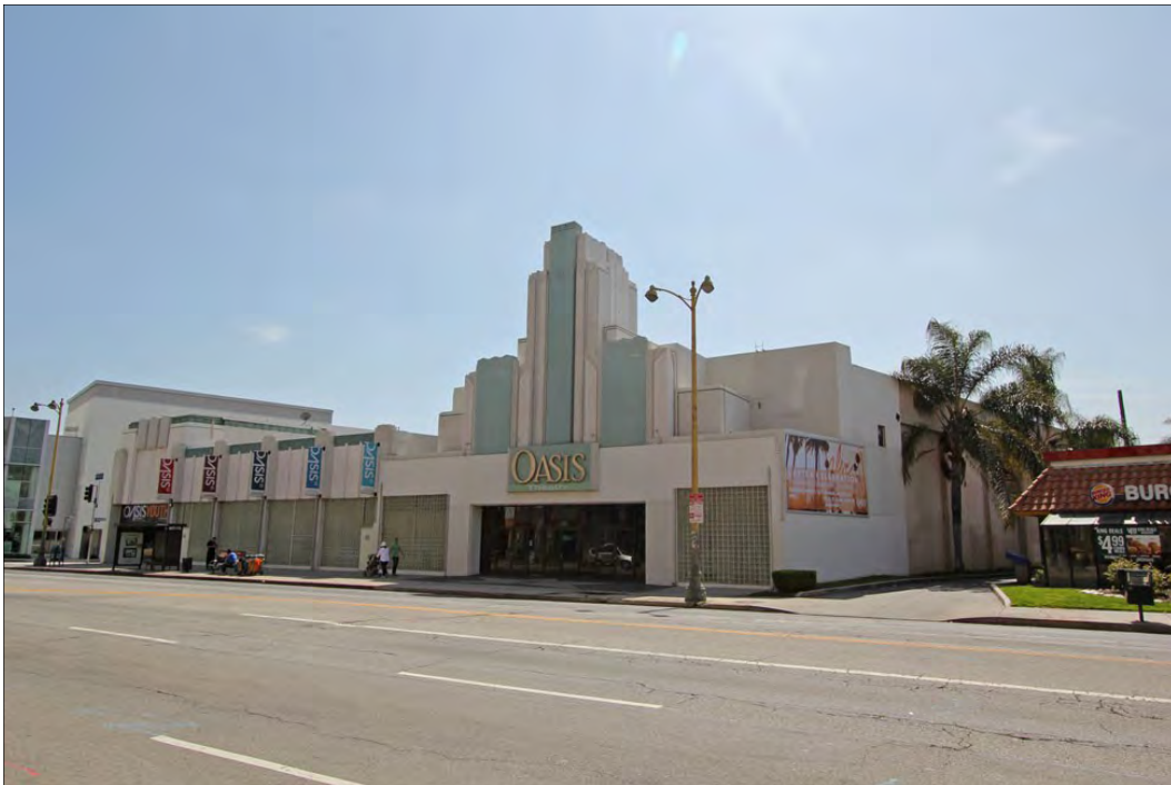
Figure 1: Main, north elevation, view southeast (Chattel, 2013)
