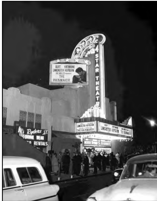
Figure 43: North façade, view southwest (Bison Archives, 1956)
