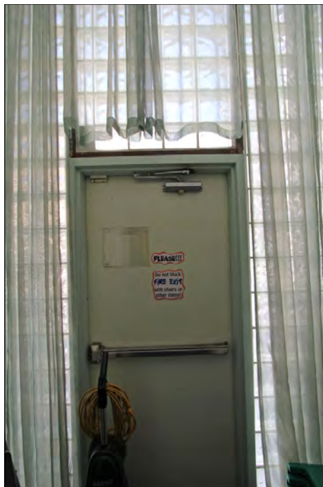
Figure 21: Typical glass block store-front in store building, view north (Chattel, 2013)
