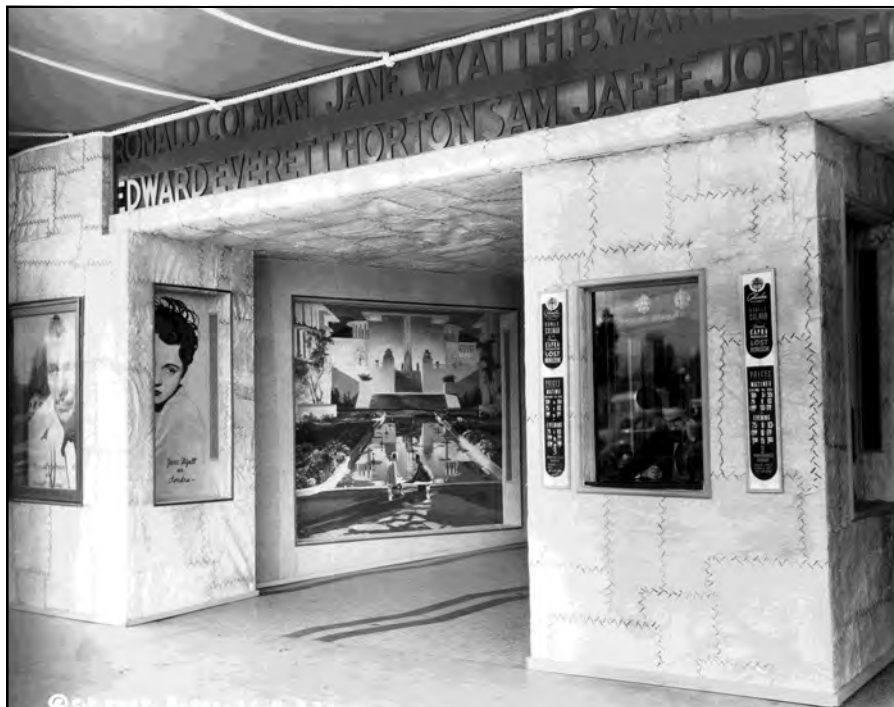
Figure 34: North façade, box office, note temporary wrapping on box office and entry for specific movie, view southeast (Bison Archives, 1937)
