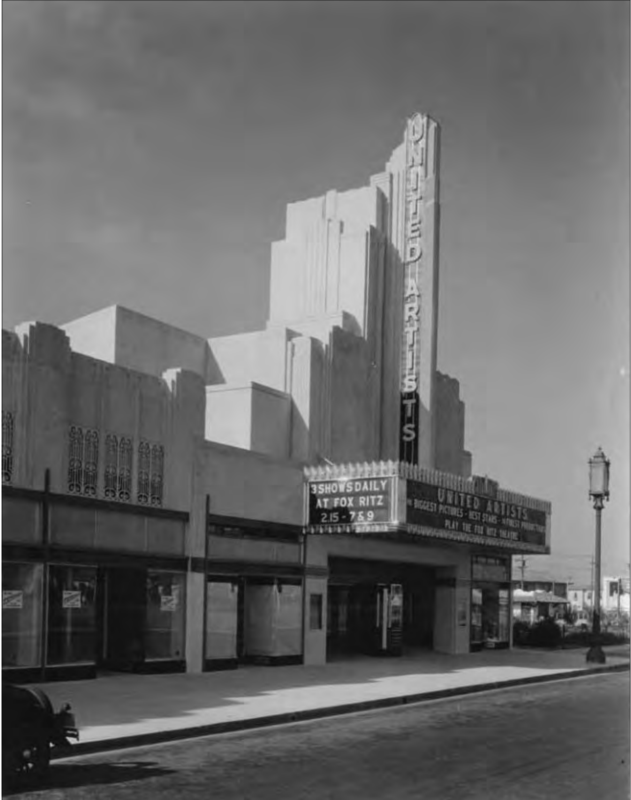
Figure 28: North façade, view southwest (California State Library, Mott Studios, c.1932)
