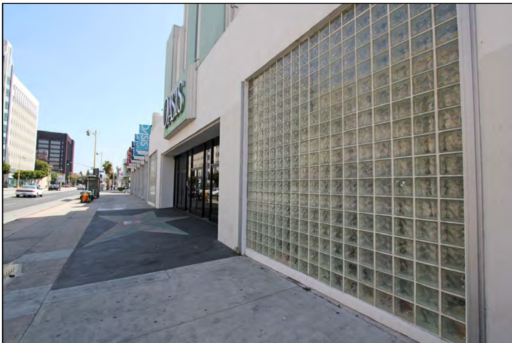
Figure 4: North elevation, main entrance, view east (Chattel, 2013)
