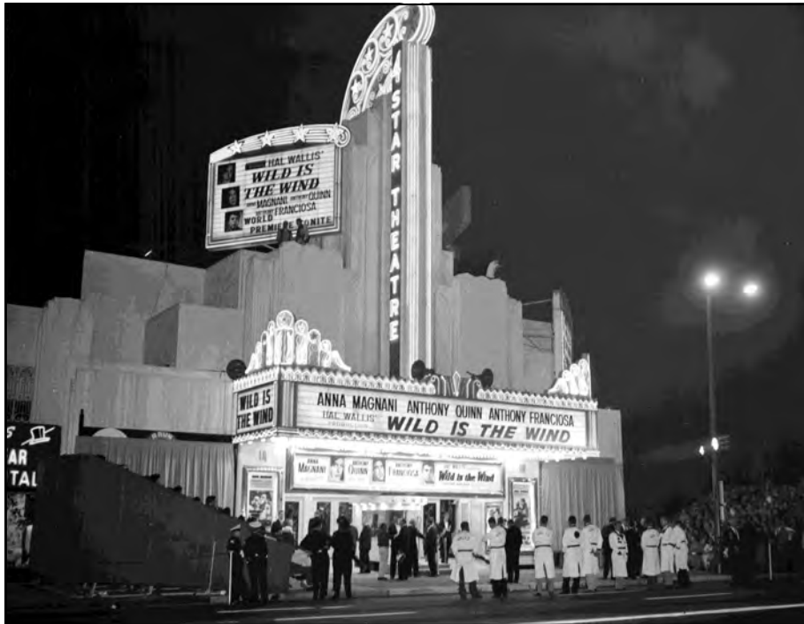
Figure 45: North façade, view southwest (Bison Archives, 1957)
