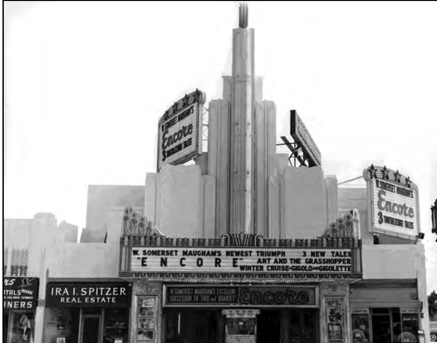
Figure 42: North facade, view south (Bison Archives, 1952)
