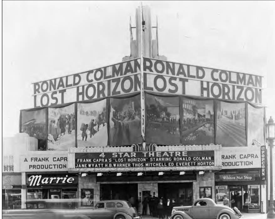
Figure 32: North façade, view south (Los Angeles Public Library, 1937)
