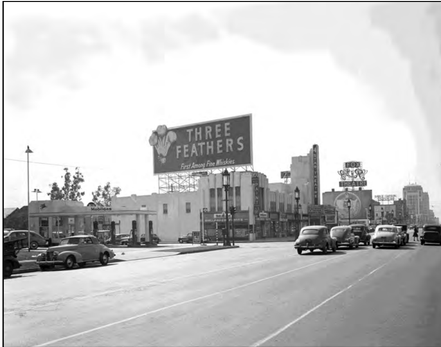
Figure 39: West elevation (left) and north façade, view southwest, note blade sign with four stars (Bison Archives, 1946)
