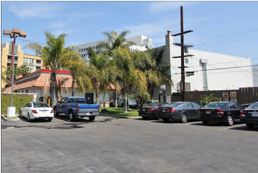
Figure 9: Rear, south elevation, from across parking lot of adjacent parcel, view north-east (Chattel, 2013)
